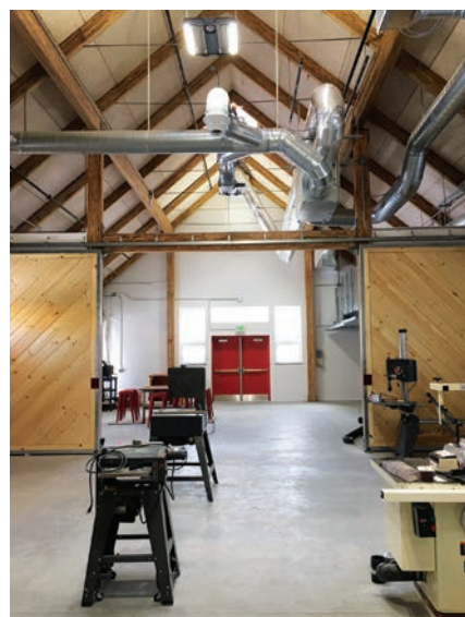
Inside view of the Bente Torjusen West Sculptural Studies Building
